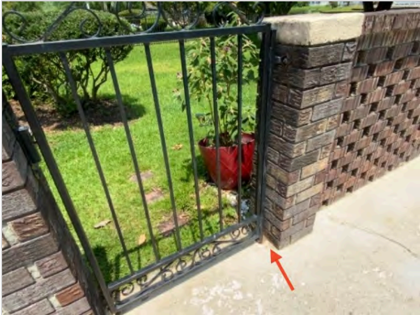
Left gate not attached.
